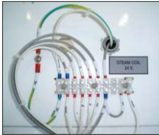
Figure.3-14 Steam Valve Connection
